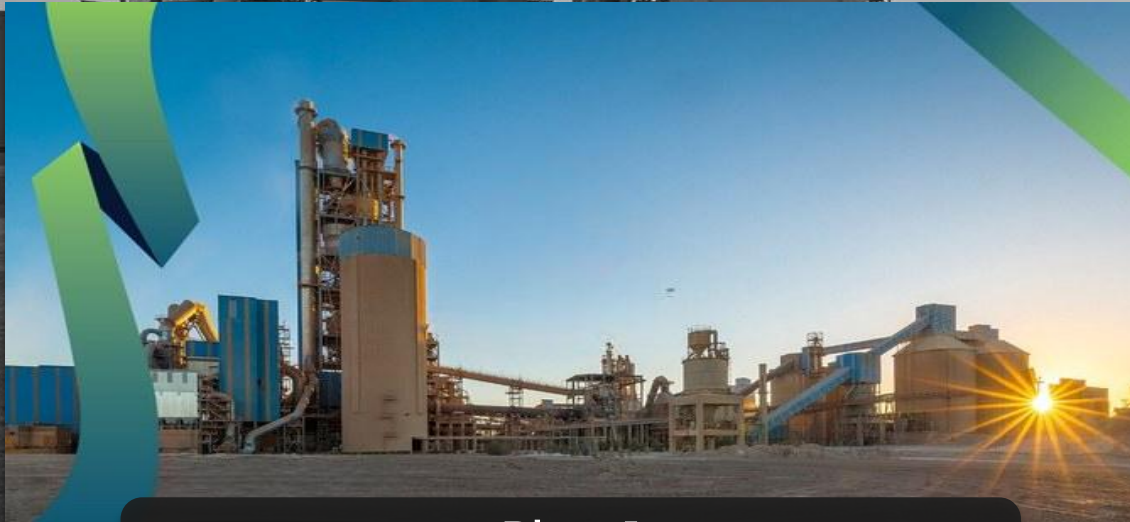
Plant 1 Buraidah – Qassim Region
